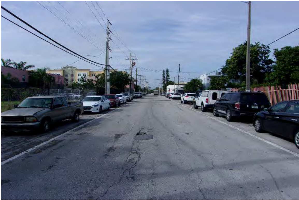
LOOKING WESTERLY ON N. W. 7 TH STREET – SUBJECT TO LEFT
