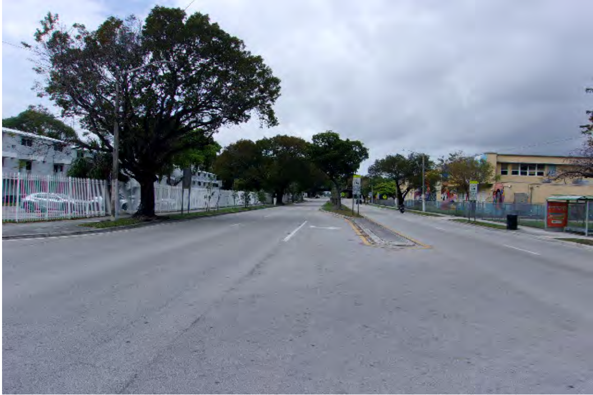
LOOKING WESTERLY ON N.W. 20 TH STREET – SUBJECT TO LEFT
