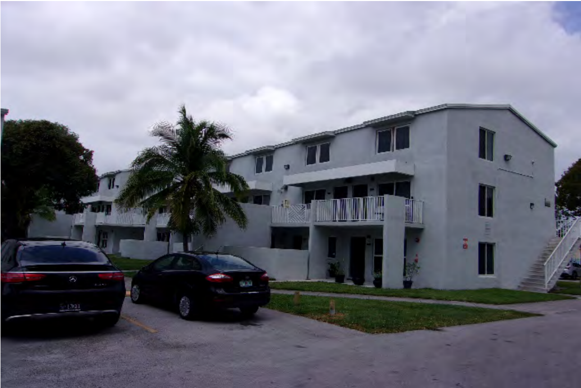
LOOKING NORTHWESTERLY AT SUBJECT BUILDING
