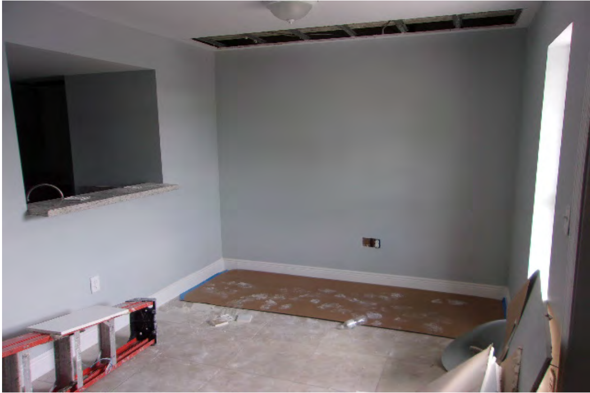
INTERIOR VIEW - SUBJECT UNIT
