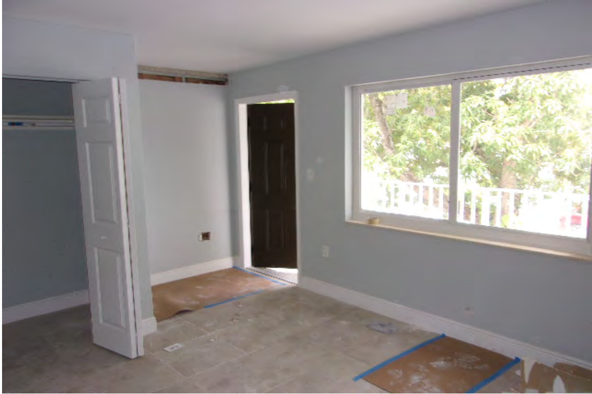
INTERIOR VIEW - SUBJECT UNIT
