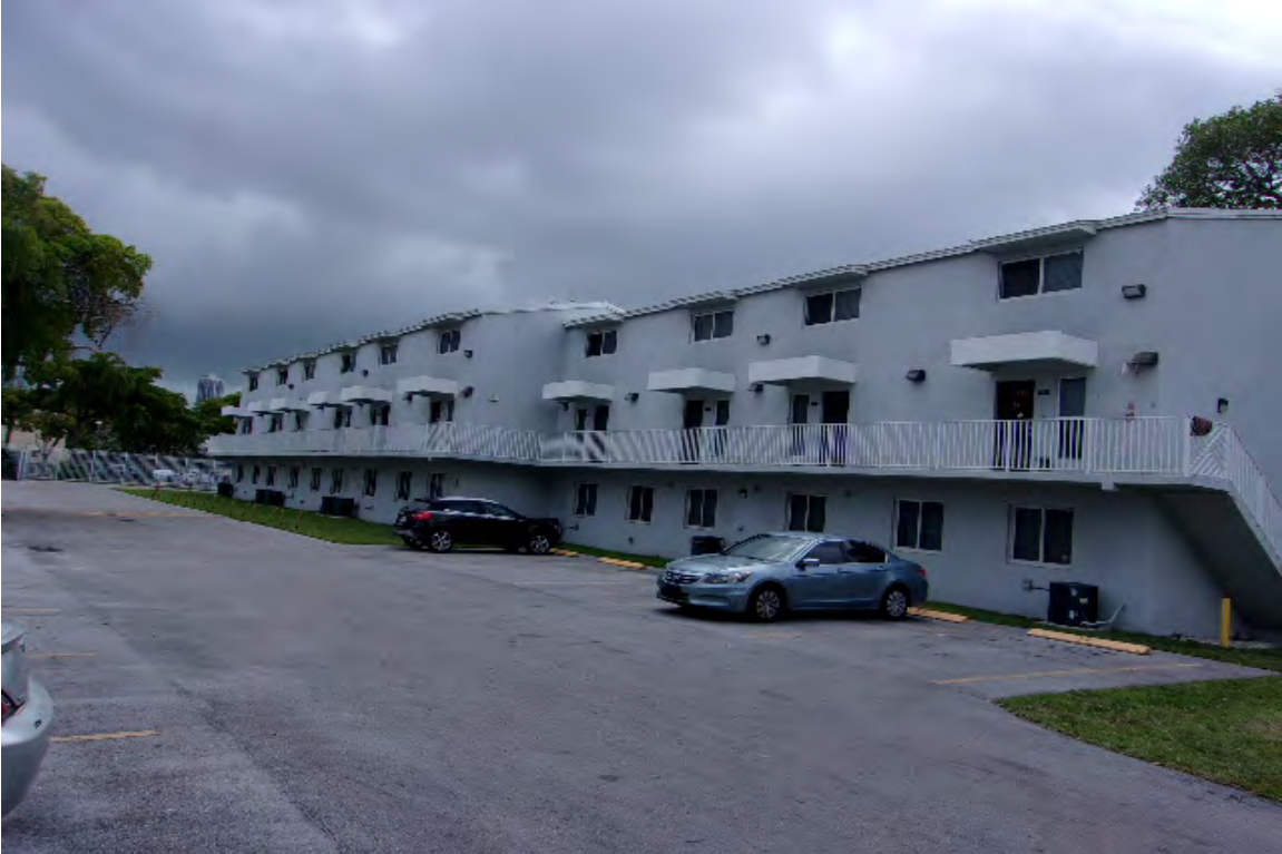
LOOKING SOUTHEASTERLY AT SUBJECT BUILDING
