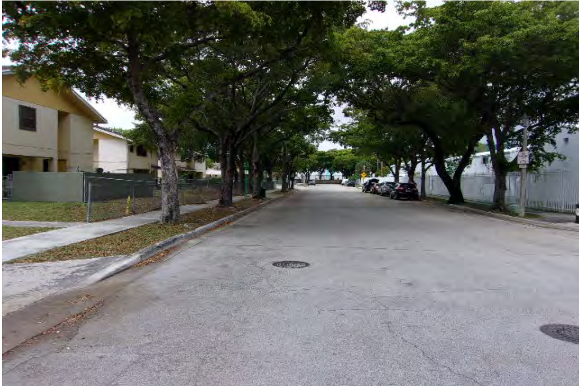
LOOKING WESTERLY ON N.W. 19 TH STREET – SUBJECT TO RIGHT
