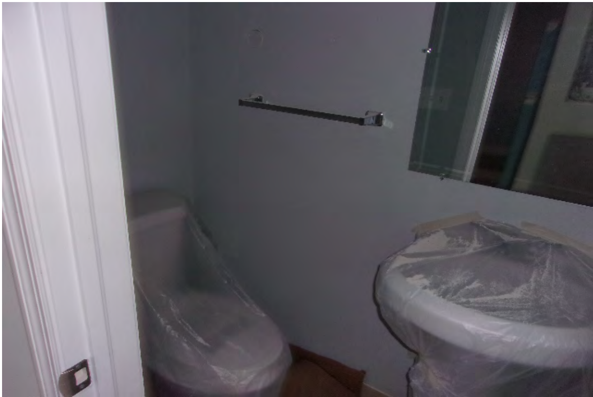
INTERIOR VIEW - SUBJECT UNIT
