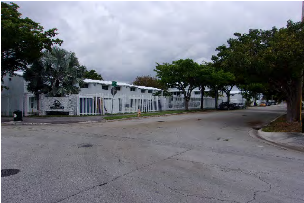
LOOKING NORTHWESTERLY AT SUBJECT PROJECT FROM N. W. 4 TH COURT
