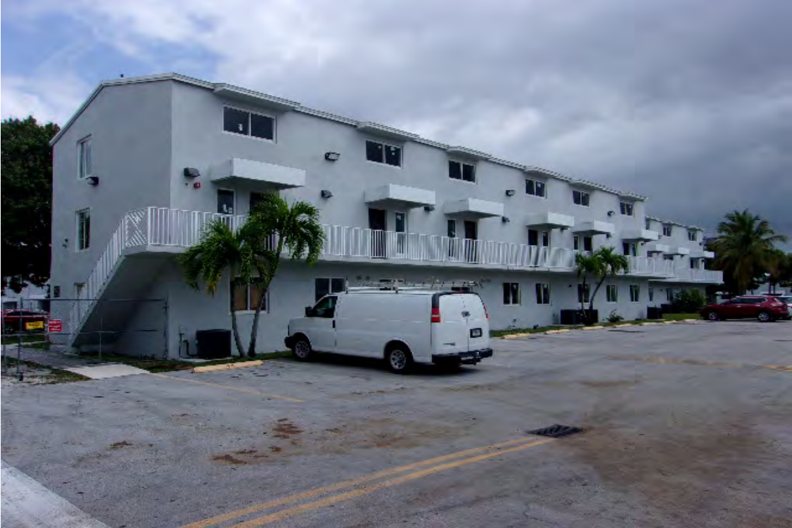
LOOKING NORTHEASTERLY AT SUBJECT BUILDING
