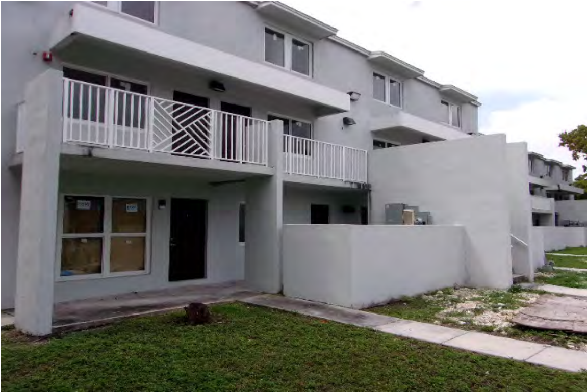
LOOKING SOUTHWESTERLY AT SUBJECT BUILDING
