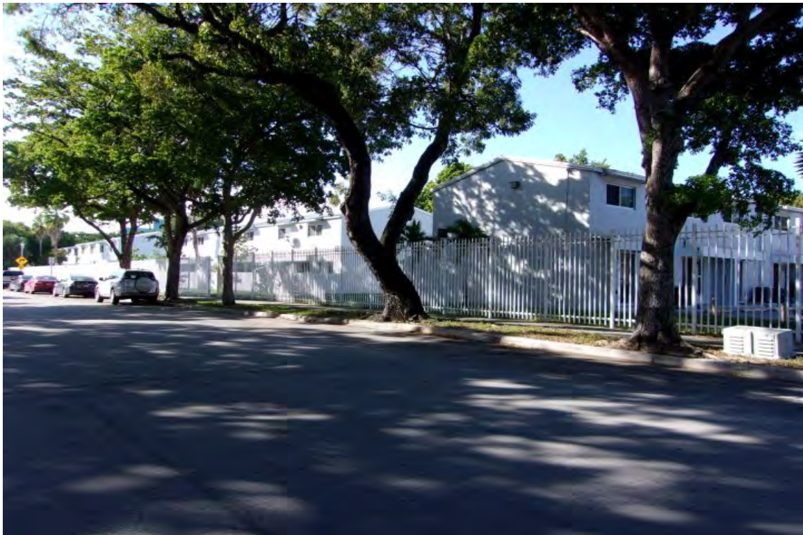
LOOKING NORTHWESTERLY AT SUBJECT PROJECT FROM N. W. 19 TH STREET
