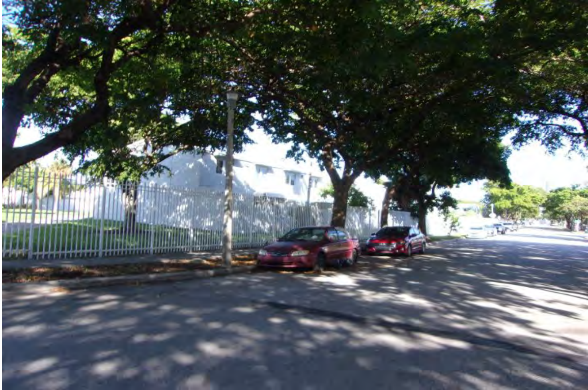
LOOKING NORTHEASTERLY AT SUBJECT PROJECT FROM N. W. 19 TH STREET
