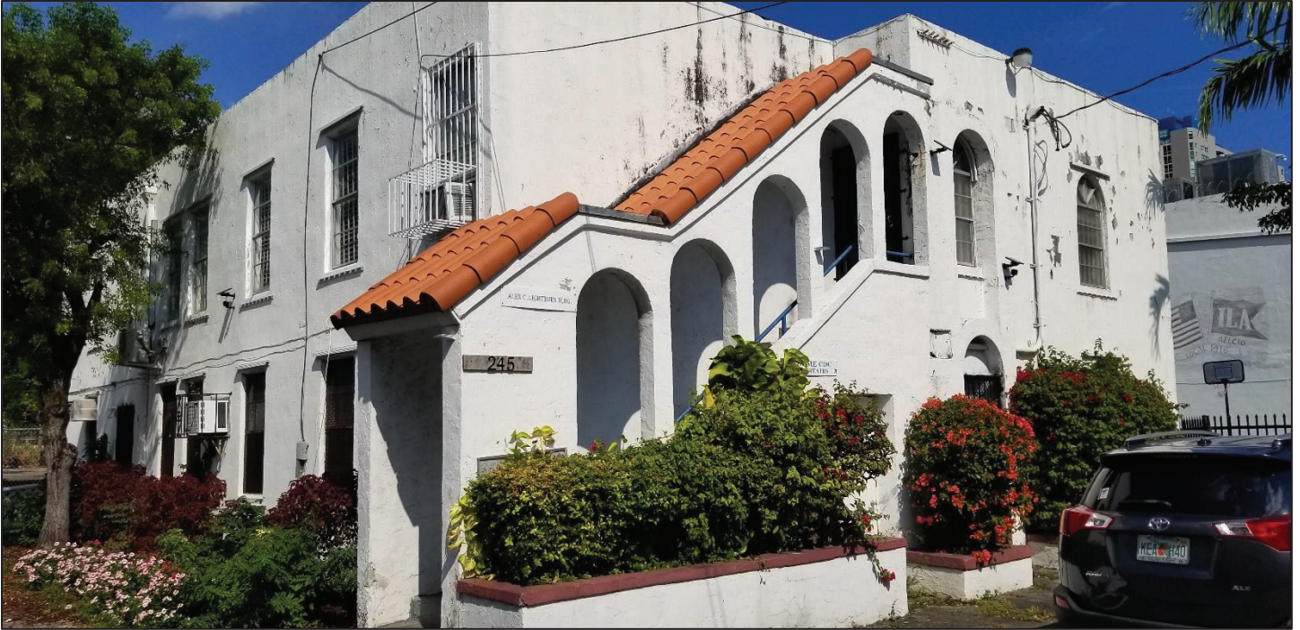
25) Smaller adjacent structure, South east view
