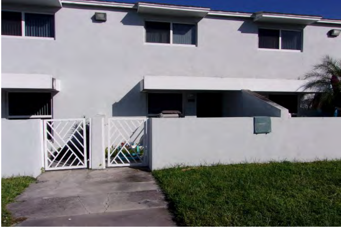
LOOKING EASTERLY AT SUBJECT UNIT
