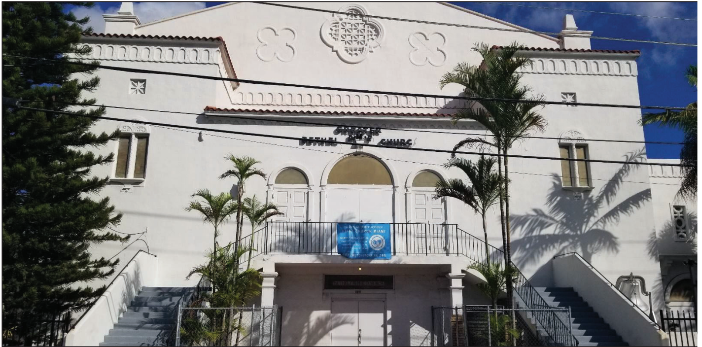
1) South Elev. view, main entrance
