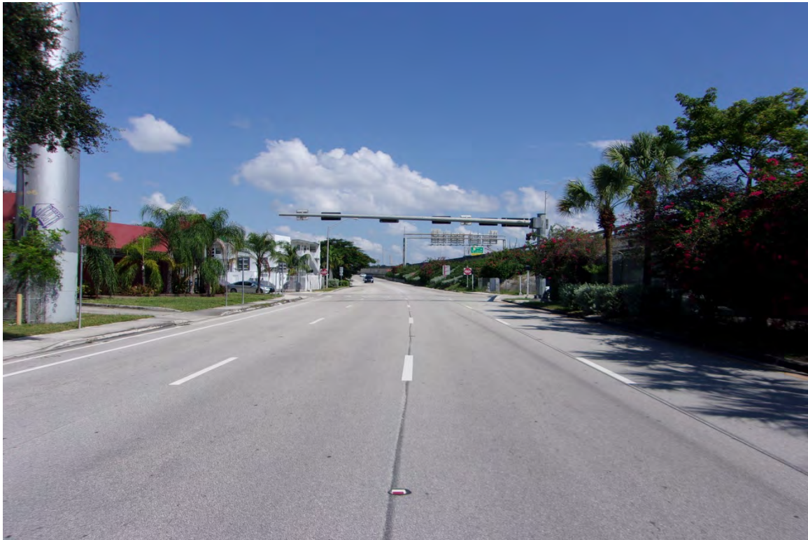
LOOKING NORTHERLY ON N. W. 3 RD AVENUE- SUBJECT TO LEFT
