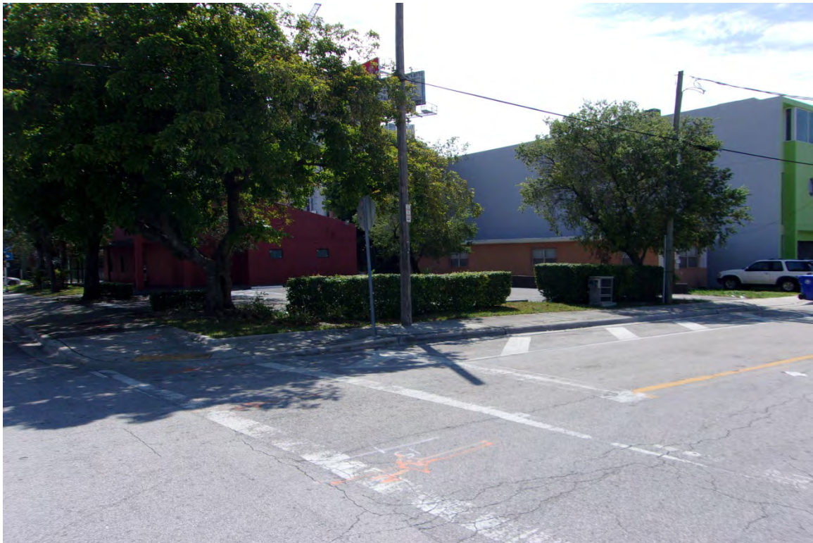
LOOKING SOUTHEASTERLY AT SUBJECT FROM N. W. 4 TH AVENUE
