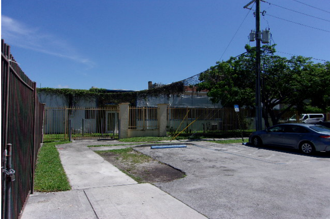
LOOKING NORTHEASTERLY AT PARCEL 3 FROM N. W. 13 TH STREET
