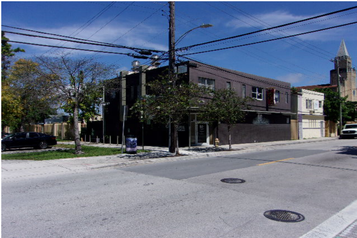
LOOKING NORTHWESTERLY AT PARCEL 1 FROM N. W. 3 RD AVENUE
