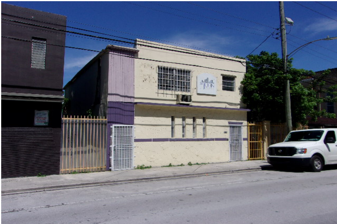
LOOKING NORTHWESTERLY AT PARCEL 2 FROM N. W. 3 RD AVENUE
