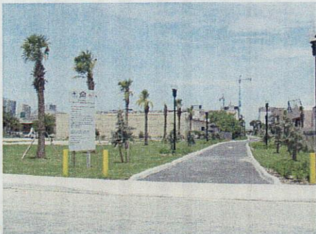
Grand Promenade Interim Renovation Project- July 12, 2005.
